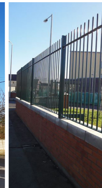
Southern boundary with Scholarstown Road - Existing boundary wall will be lowered and finished with brick and granite coping with black metal railing.
