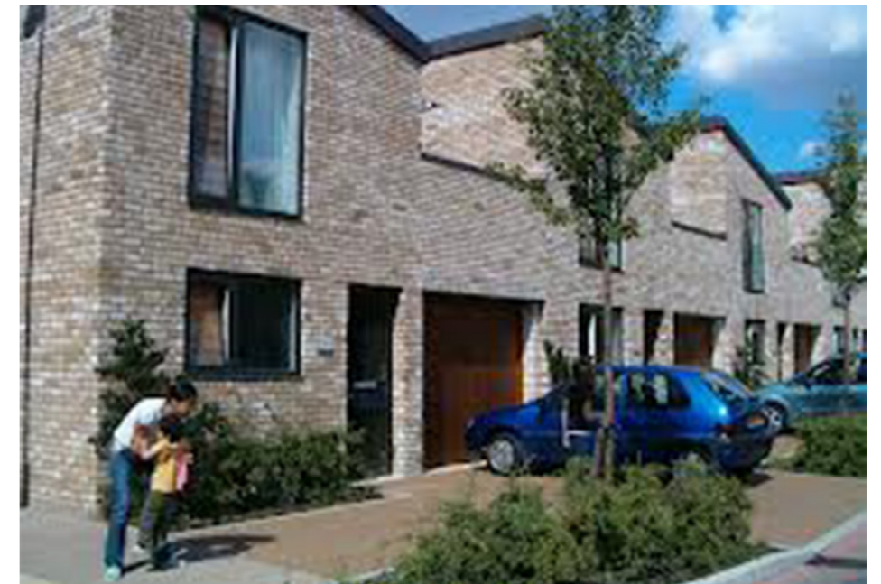
Paving for the dwellings’ ‘doormats’: tegula PC block paving ( www.tobermore.co.uk sizes: 173 x 173 x 80mm
